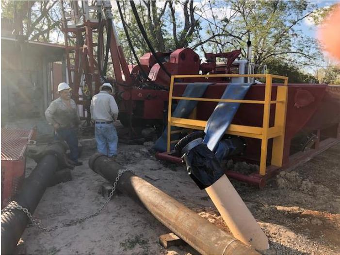
**Figure 3: Piping Used For Acidization and Jetting of Well 19**
